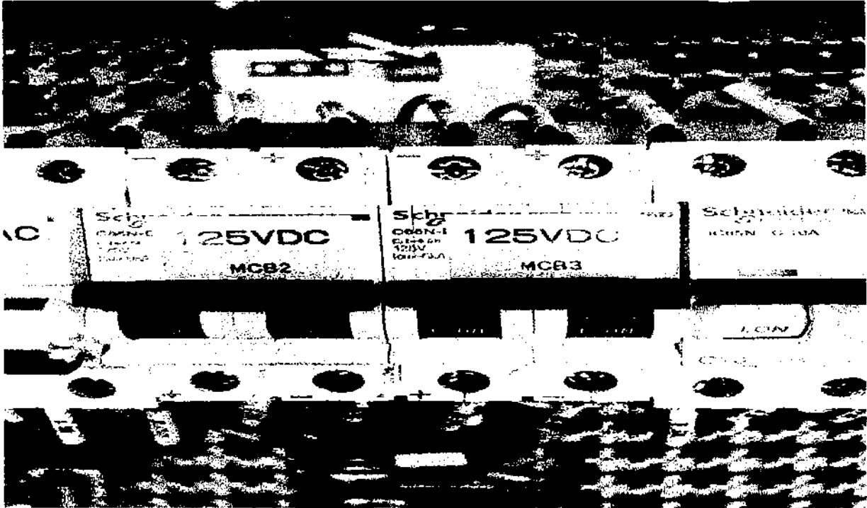
Item no. 3 Breaker, ICN65N – 125VDC, 6kA, 2-Poles
